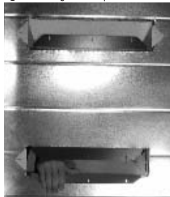
figure 2.3b - Unfold the ducting flairs completely to sandwich the return air plenum between the ducting flairs and the filtration unit.
