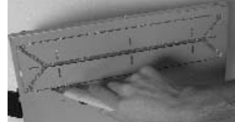
figure 2.2a - Cut the insulation along the inside edge of both inlet and outlet ports to remove the insulation from the port openings.
